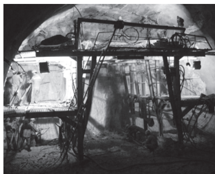
Carmel Tunnels, Drilling holes for blasting
