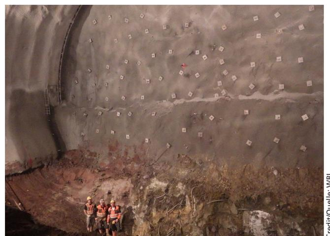
10 Heading central station south, excavation of invert area
